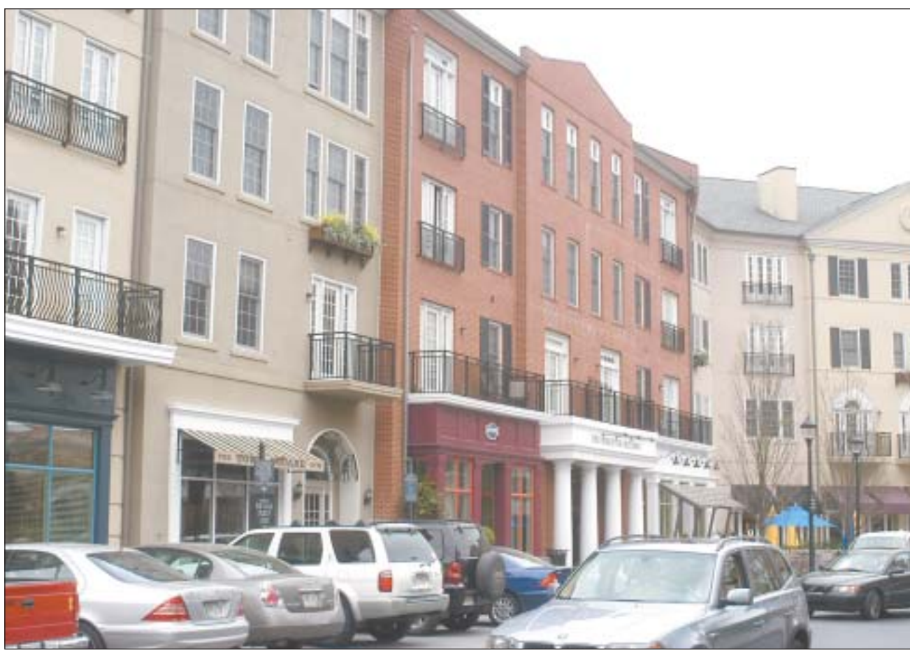
Post Riverside, an apartment complex in Atlanta, Ga., was designed by Andres Duany, creator of the SmartCode. Riverside feels like a traditional European city. Multi-level apartments are built around a typical town square, and retail shops and restaurants occupy the first floor. The public area accommodates both pedestrians and vehicular traffic.
