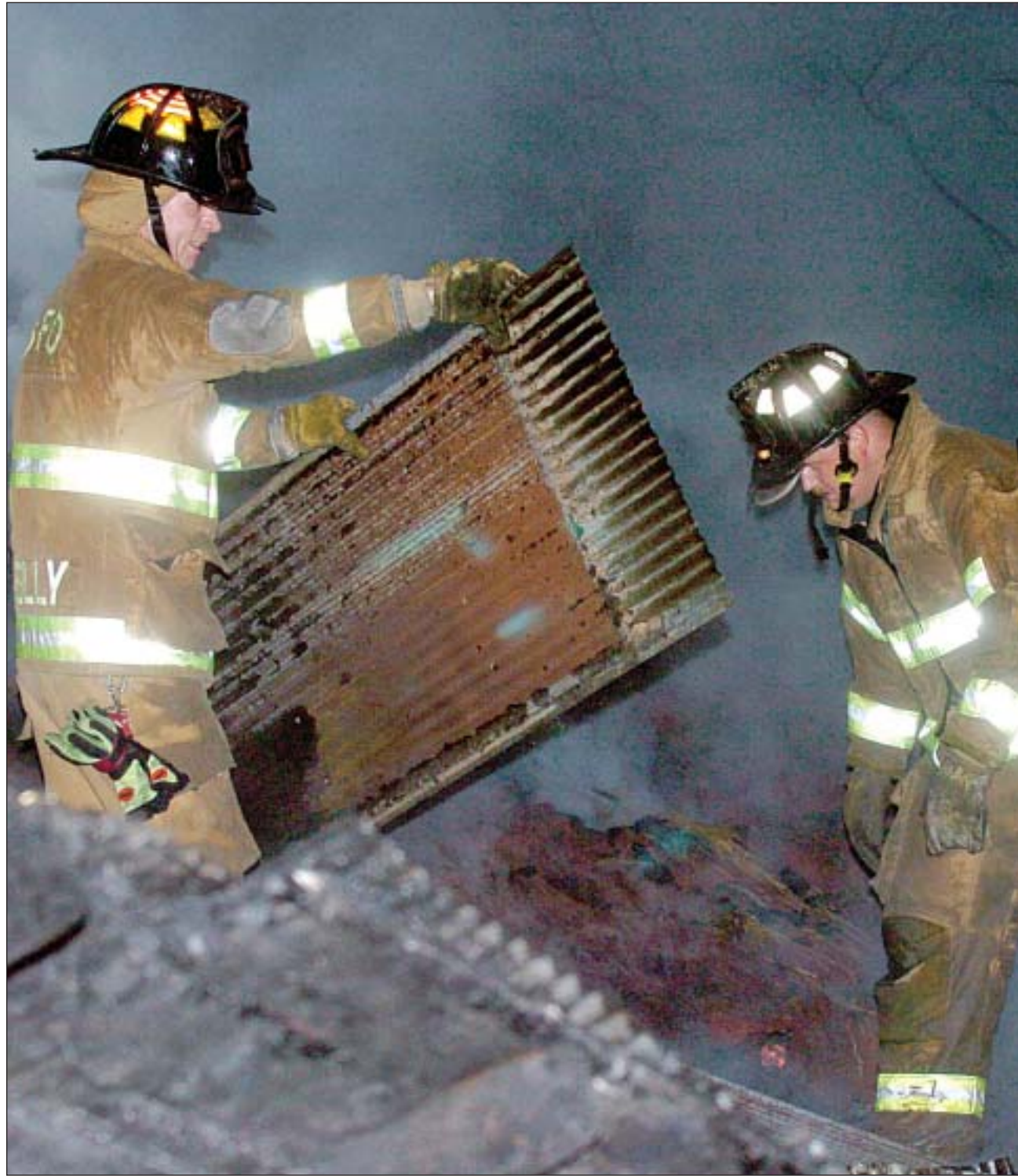
After dousing the fire Bentonville firefighters worked to remove the tin roof of a hay barn in the early morning hours of Saturday near the intersection of Southwest Elm Tree and Southwest Eighth Streets in Bentonville. The fire was believed to have been caused by lightning. No injuries were reported.
