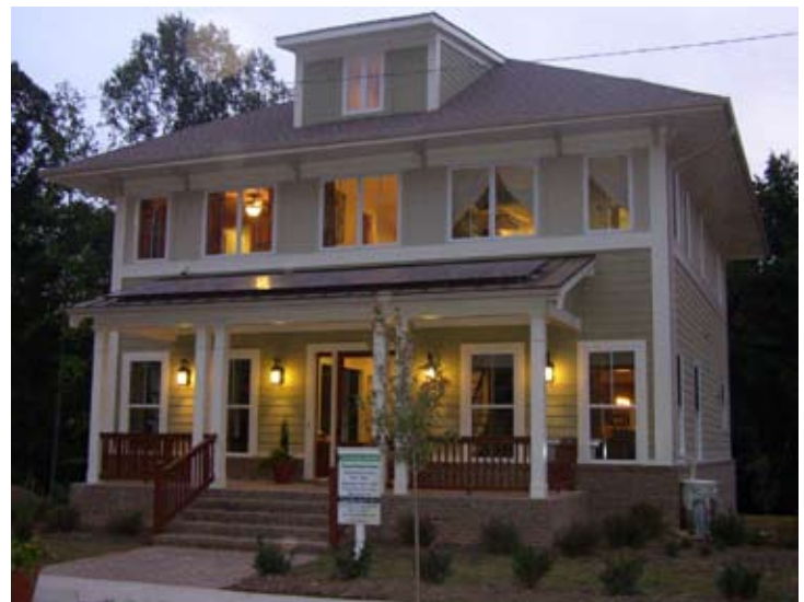
Top: Sketch elevation of Going Green House Above: Completed Going Green House
