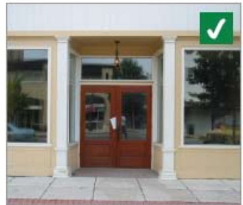
Primary pedestrian entrances recessed a maximum of 7 feet from the exterior facade.
